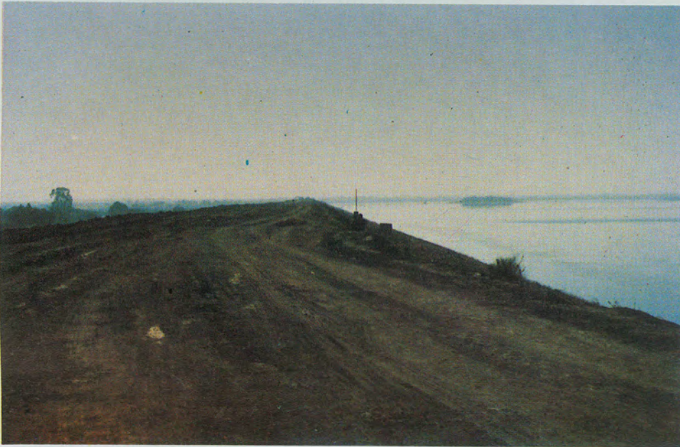
VIEW OF GALWA RESERVOIR
