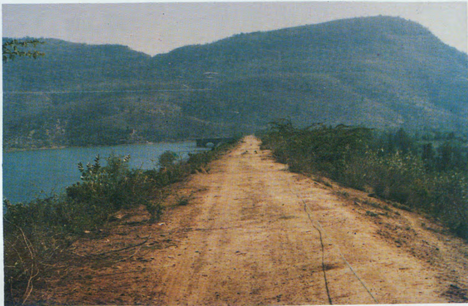
VIEW OF MANSAROVAR RESERVOIR
